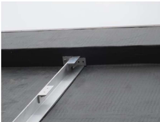
Top Left - Top and only penetration mechanically fastened
