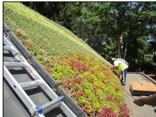
Green Living Wall; Sloped Green Roof - Pre-Grown Installation- NON-Penetrating Detail
