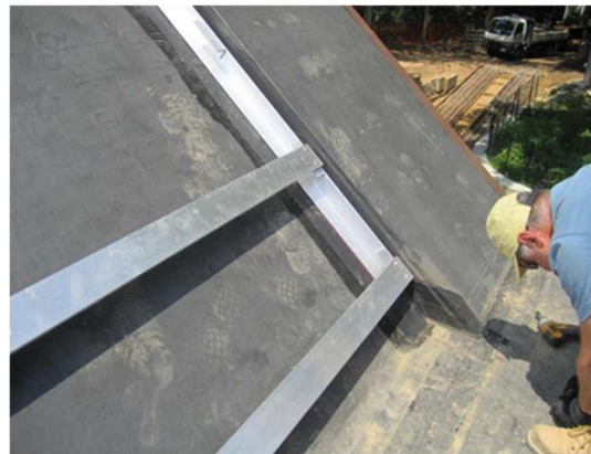
Top Right - Horizontal Supports to the vertical L bracket
