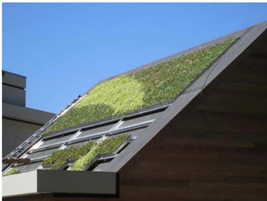
Green Living Wall; Sloped Green Roof - Pre-Grown Installation- NON-Penetrating Detail
